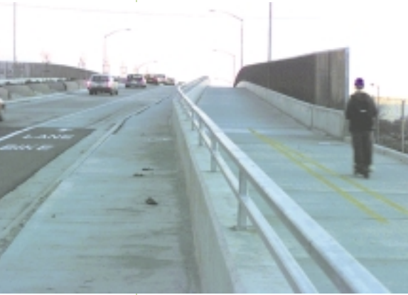
Figure 25. Shared Use Path (Far Right) on a Grade Separation Structure; Note Bike Lane and Sidewalk.
