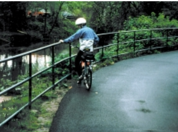
Figure 18. Safety Rail Between Shared Use Path and Adjacent Slope and Waterway
