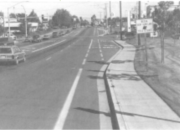
Figure 9. Markings for Bike Lane Merge in Advance of Intersection
